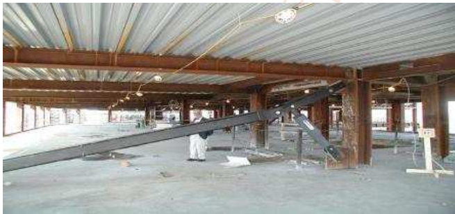
Figure2 FVD as a toggle brace element
