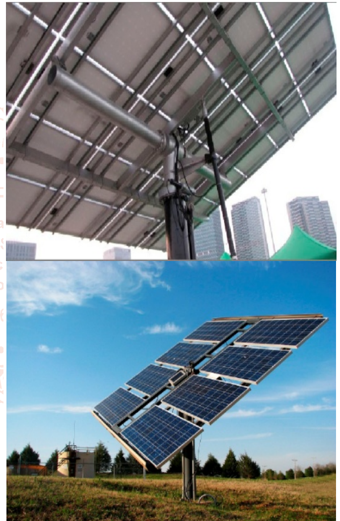
Figure 2. A solar photovoltaic station with a two-axis tracker.
