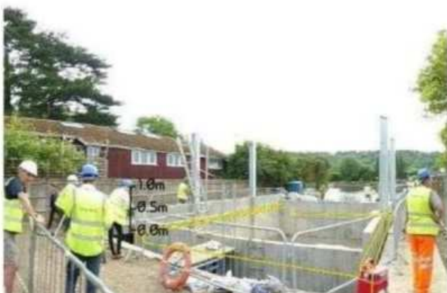
Fig - 4: Construction of amphibious house
