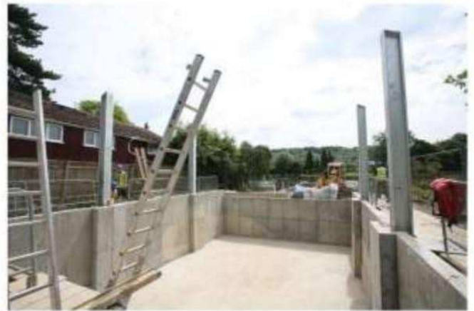
Fig – 5: Construction of amphibious house
