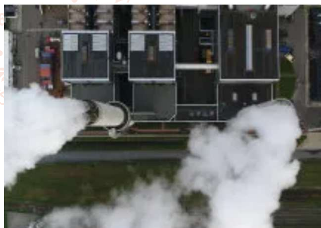
Fig. 2.4 CO 2 Emission from Cement manufacturing Plant Causes Air pollution.
