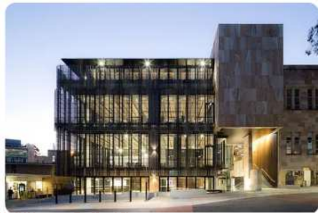
Fig. 3.2 A Building made by the Geopolymer Concrete [source: google images]
