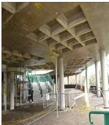
Figure 1.3 Ribbed Slab
