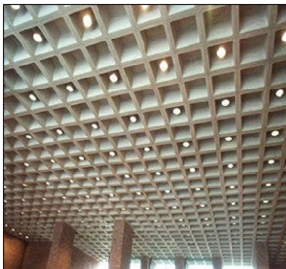
Figure 1.2 Waffle Slab
