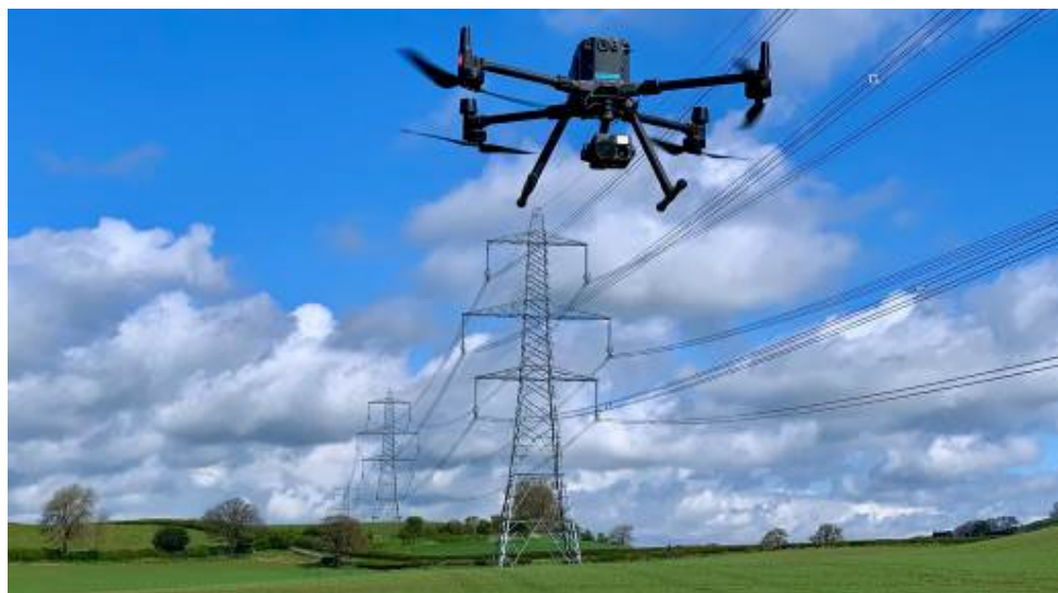
Figure 5 A drone for inspecting the national grid [8].
